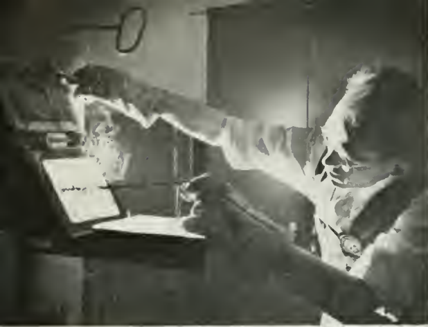
RESULTS OF WAR-TIME RESEARCH IN RCA LABORATORIES POINT TO NEW PEACE-TIME RADIO SERVICES. HERE, EXPERIMENTAL TUBE PARTS ARE BEING REMOVED FROM A HYDROGEN FURNACE.
